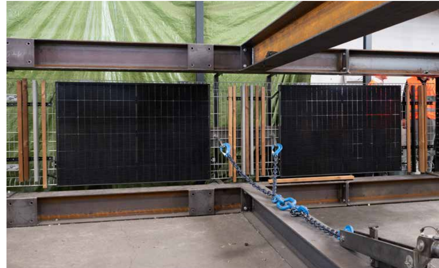
Test station with PV modules
