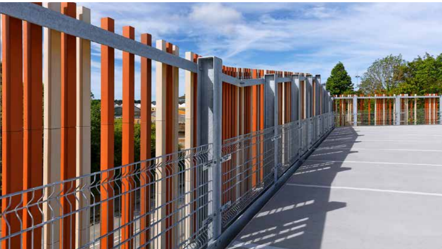
INTEGRA-pw 3.0 – Eckernförde, multi-storey car park Noorstraße
