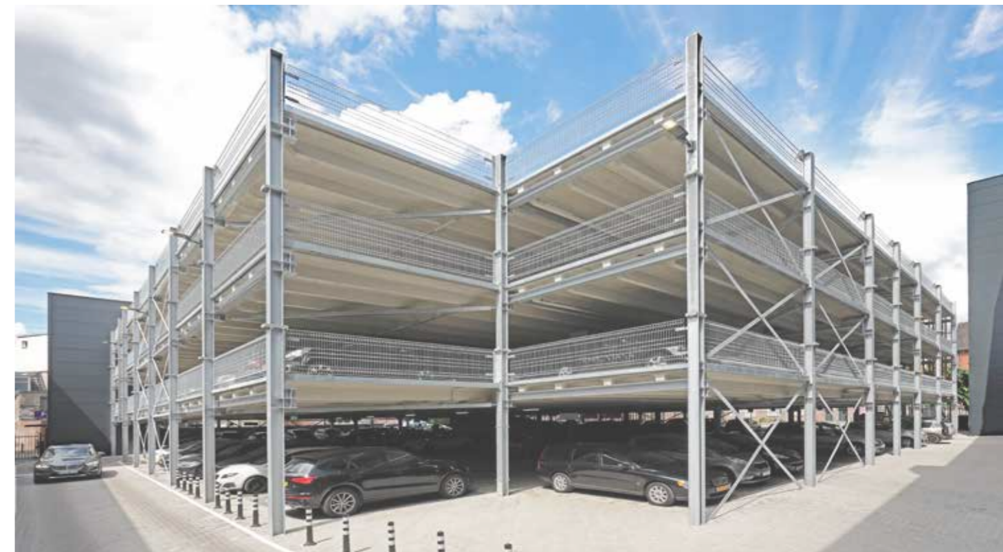
INTEGRA-pw 2.5 – Eindhoven, multi-storey car park Arsenal
