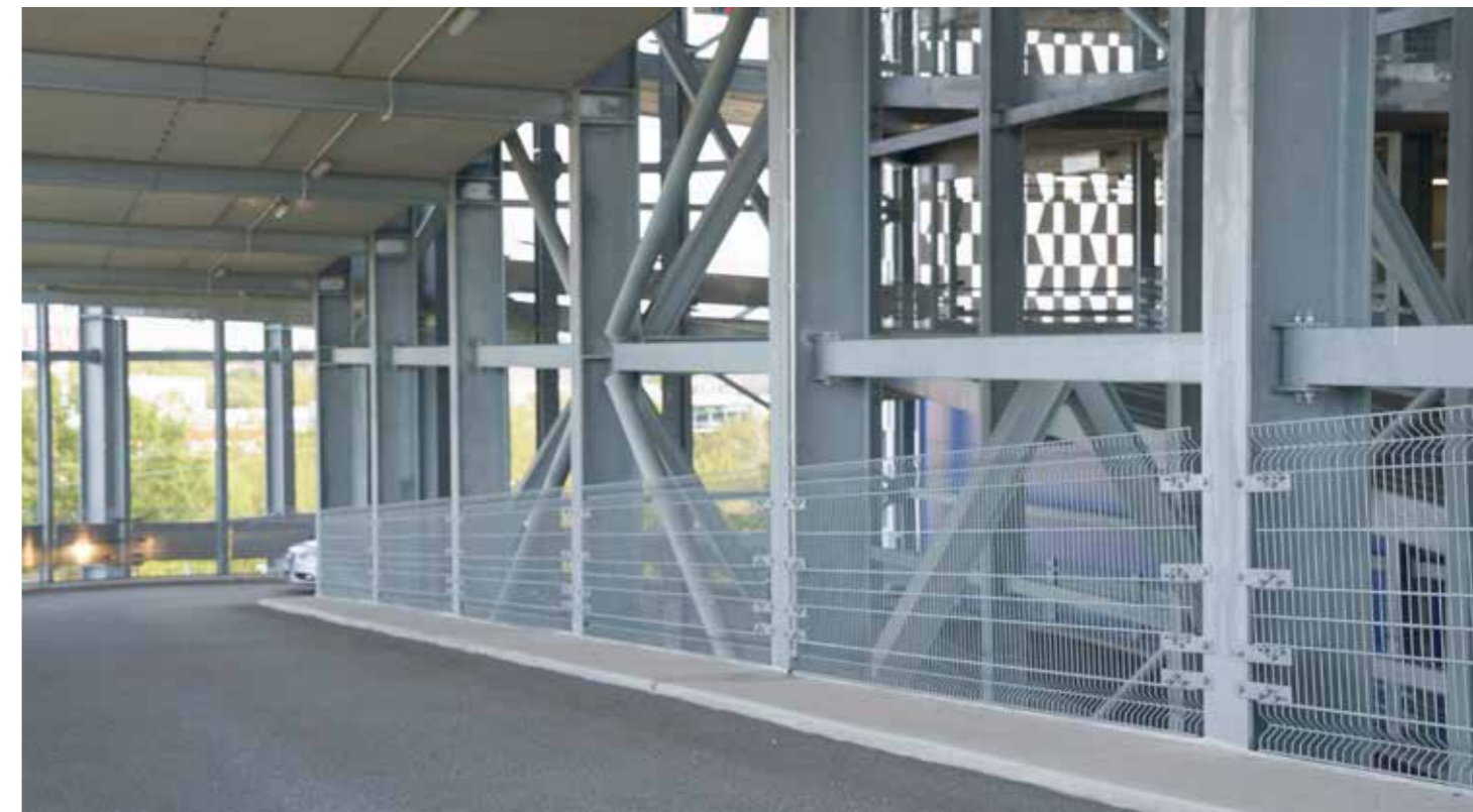
INTEGRA-pw 3.5 – multi-storey car park Furniture store
